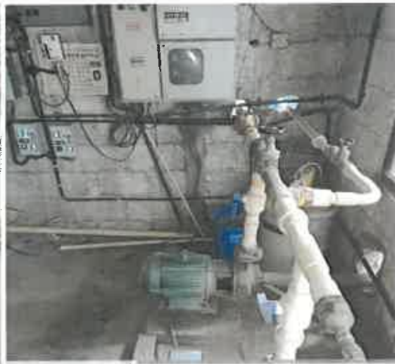
Water Station Control Board – level control and pump control
