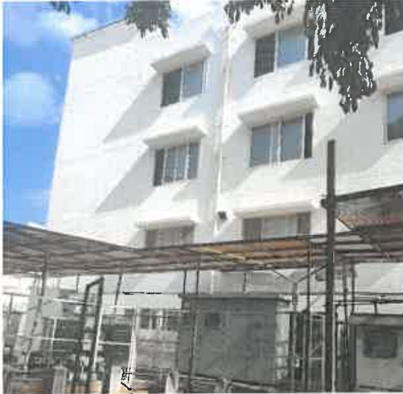
Rainwater Harvesting – Pit
