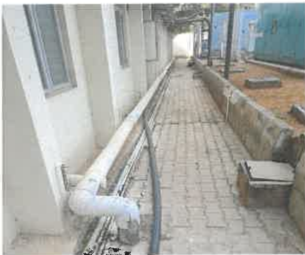
Rainwater Harvesting – pipelines
