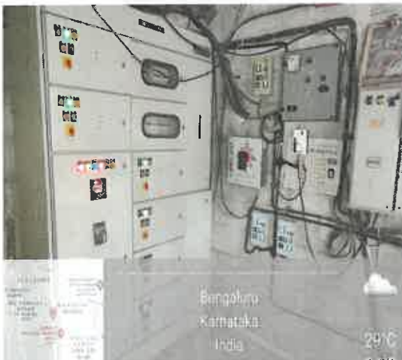
Water Station Control Board – level control and pump control
