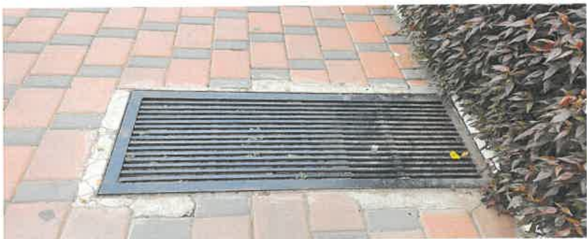
Open Rain water channels
