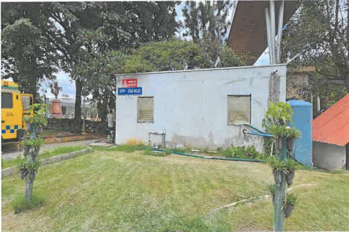
250 KLD STP at GG Campus
