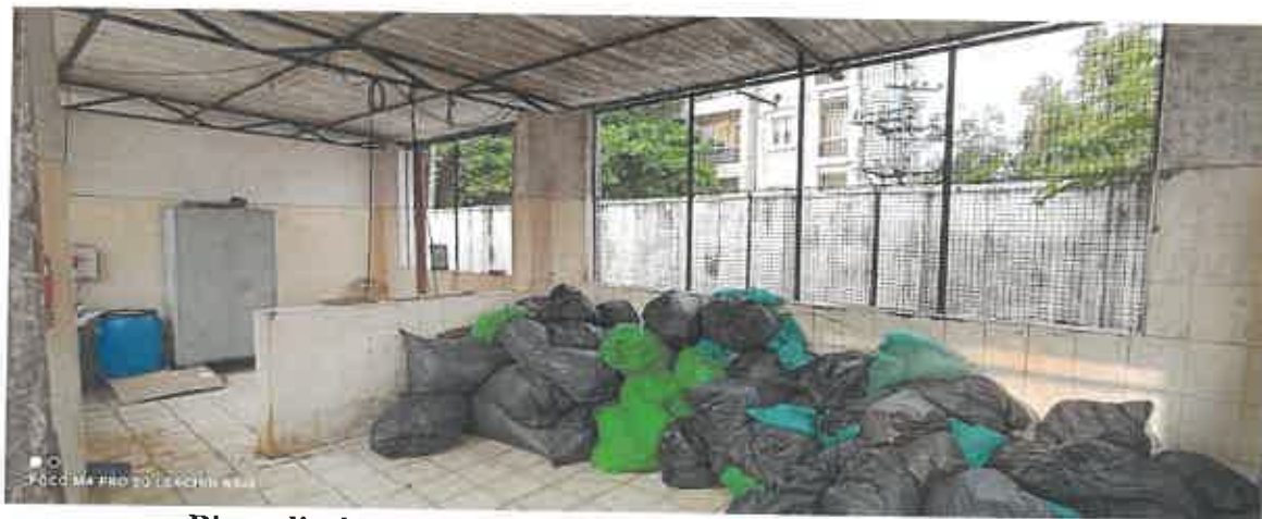
Biomedical waste segregation and storage area at GG Campus
