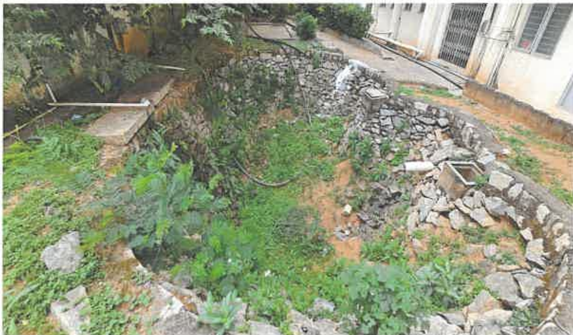
Rain water Recharge Pit
