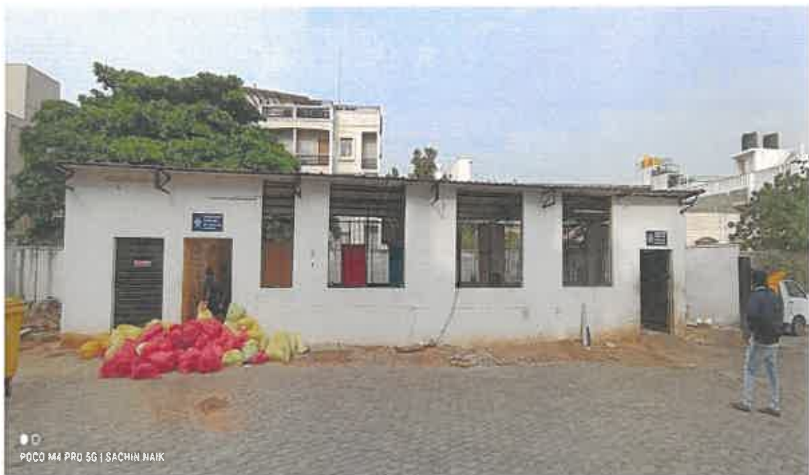
Hazardous waste room at GG campus
