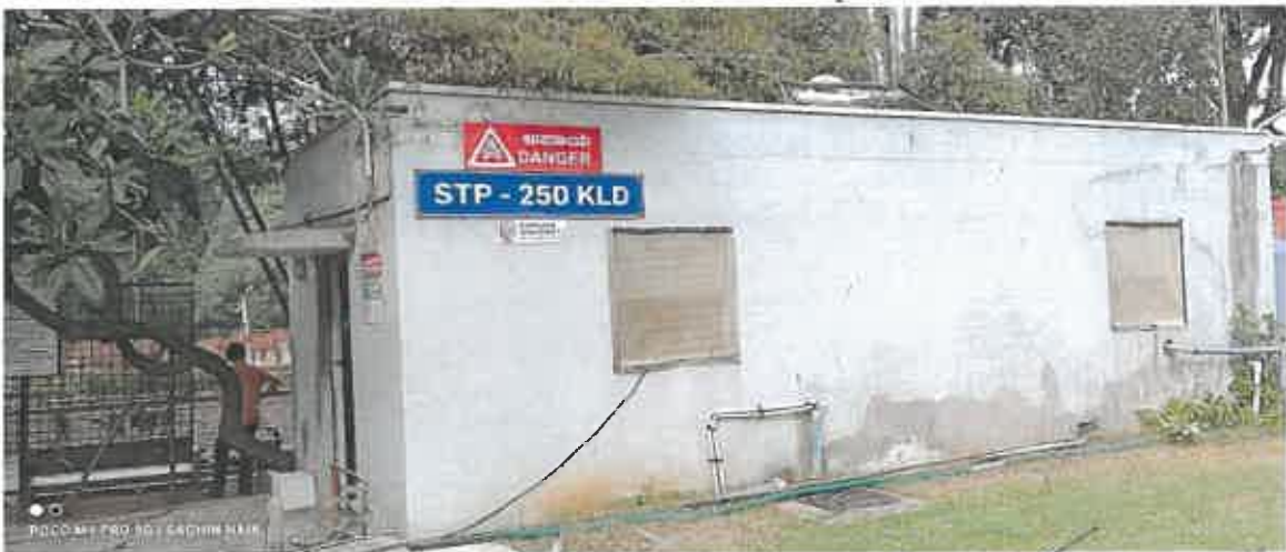
250 KLD STP at GG Campus
