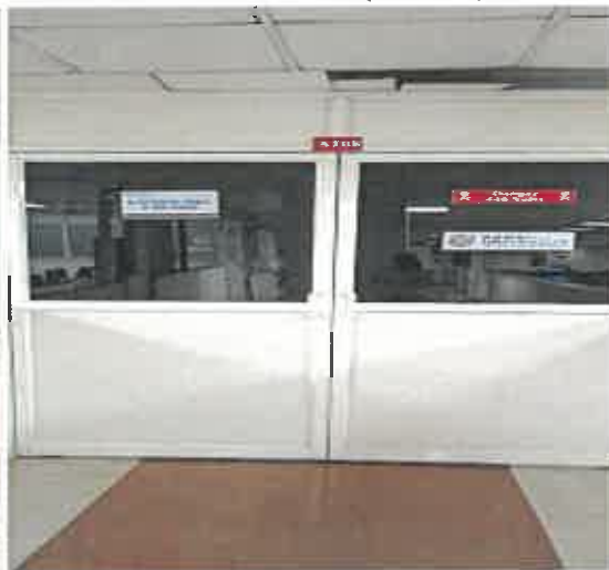
A Block UPS Room
