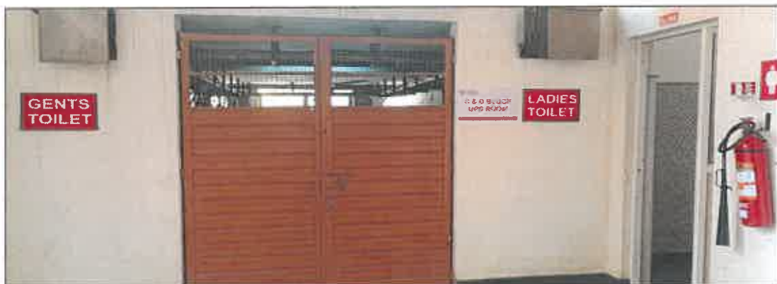
C & D Block UPS Room
